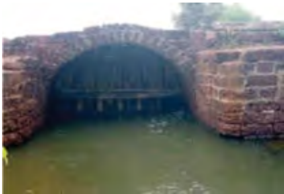
Traditional sluice gate for regulating the ingress of saline water
