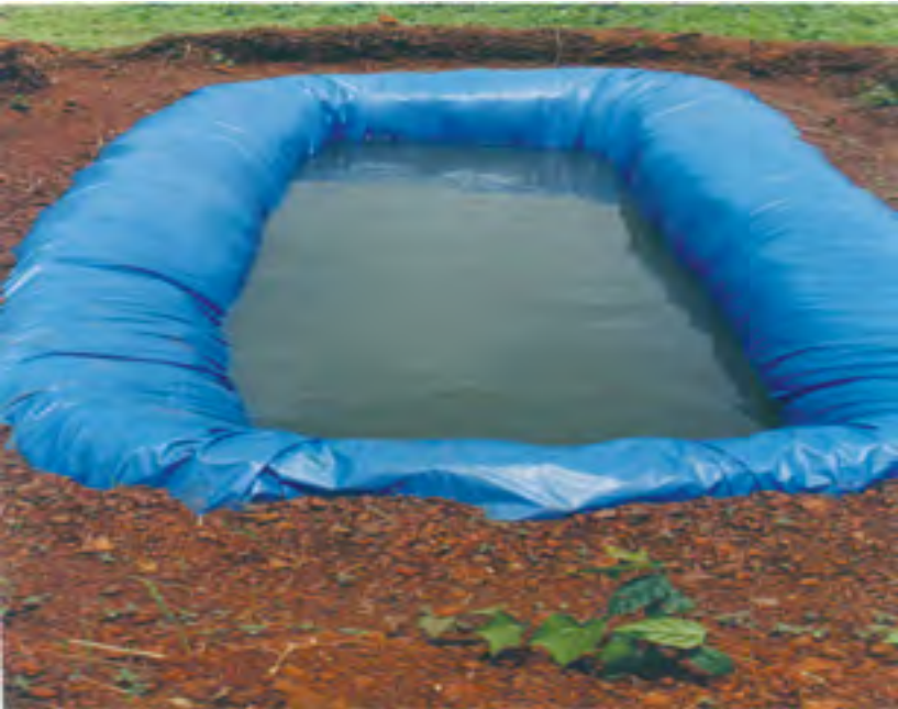
Water stored under direct water catch pits with silpaulin lining
